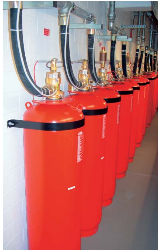
KD-200 extinguishing medium containers
